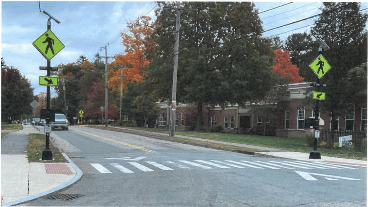
Above: Raised Crosswalk with RRFBs (Rectangular Rapid Flashing Beacons) on Main Street at Lynnfield Middle School
