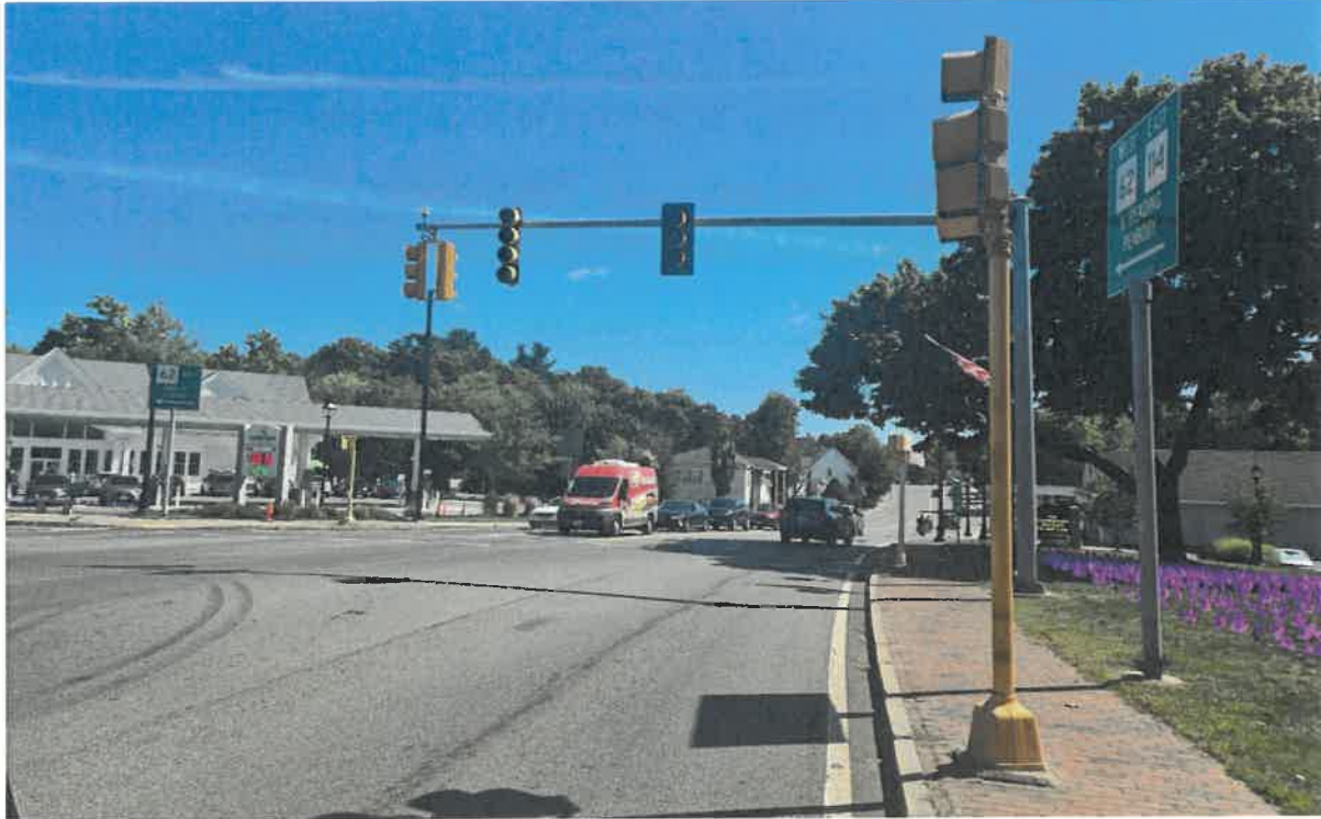
Figure 7: Signal head with prismatic lens appears dark from close-up angle
