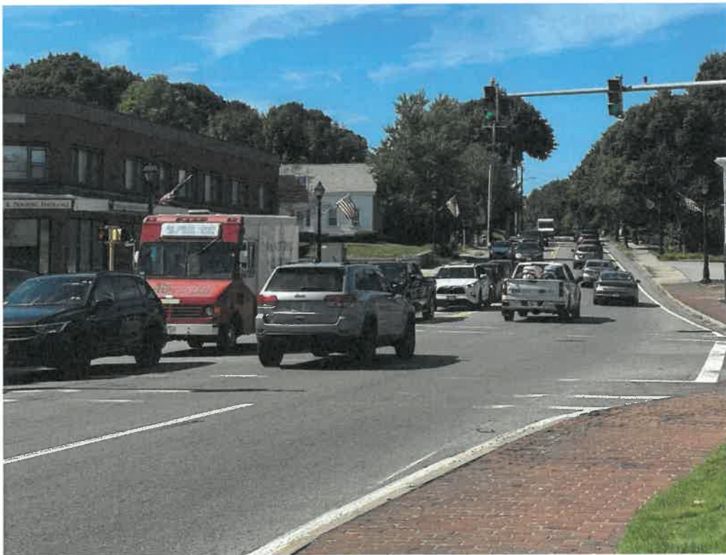
Figure 5: Faded crosswalk markings and stop bars at the Route 114/ Central Street/ Lake Street intersection.
