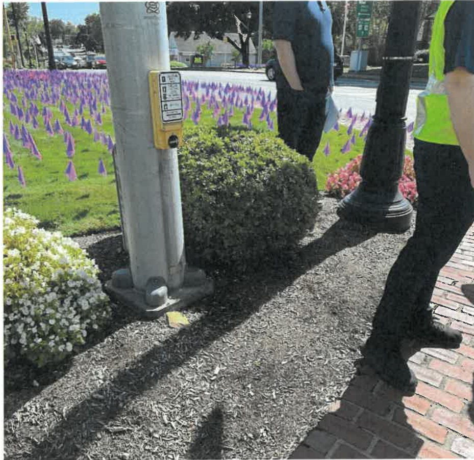
Figure 6: Pedestrian push button located out of reach of users on the sidewalk
