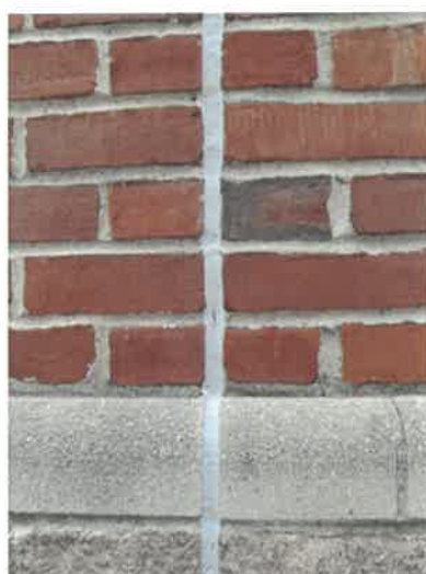
Fig. 32. Sealant material at expansion joints dried and shrinking.
