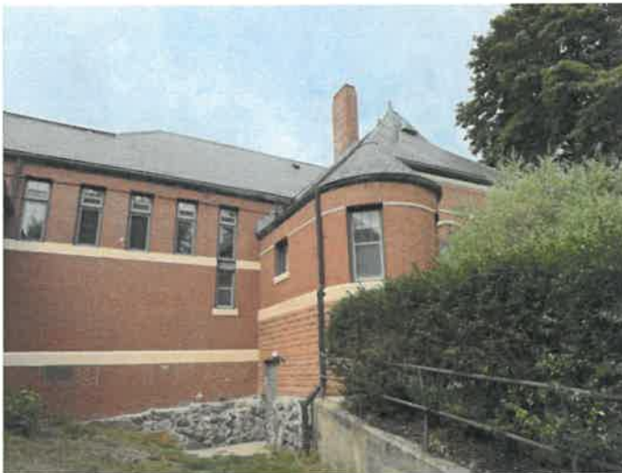
Fig. 8. Exposed granite rubble foundation wall on east elevation.
