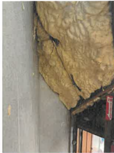
Fig. 21. Location of water infiltration at attic stairs.
