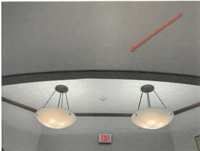
Fig. 19. Small crack in plaster over arch.
