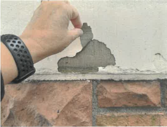
Fig. 4. Paint peeling from sandstone trim at beltcourse.
