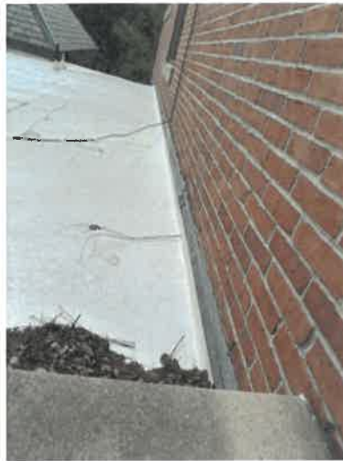
Fig. 38. Defective flashing above water leaks in Children's Library ceiling tile.
