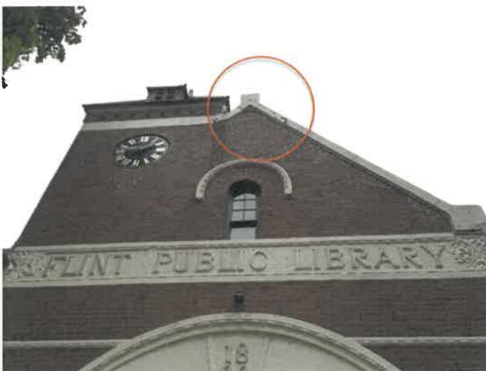
Fig. 3. Paint coating peeling from sandstone trim at gable.
