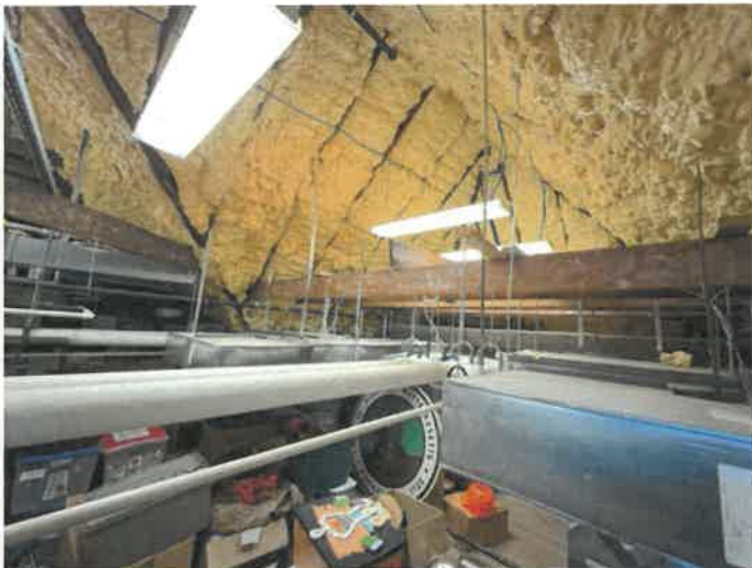
Fig. 22. Spray foam insulation installed at underside of roof.
