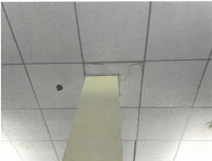
Fig. 39. Water leaks below defective flashing at flat roof above.
