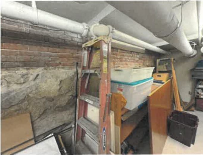
Fig. 24. Basement walls – brick and rubble stone.
