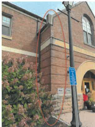
Fig. 26. Dark soiling from gable runoff.
