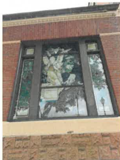
Fig. 12. Wood window trim is in poor condition, especially at the base of the mullions. Note storm windows on exterior.
