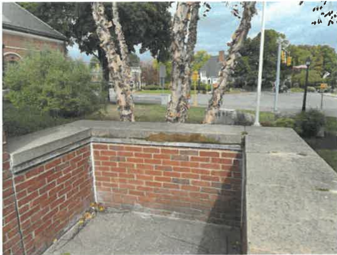
Fig. 35. Biological growth at stair capstone joints.
