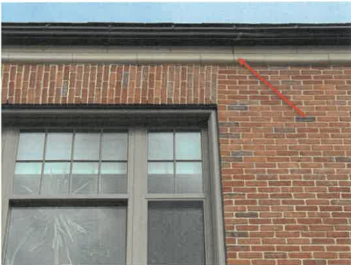
Fig. 30. Isolated cracks in cast stone.
