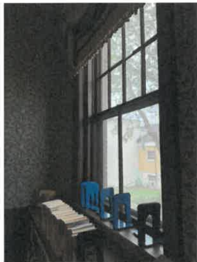
Fig. 11. Original double hung wood window.
