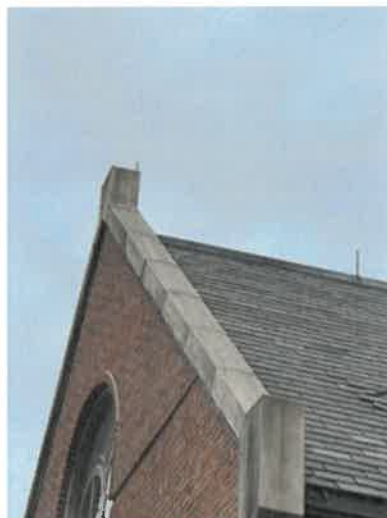
Fig. 27. Cast stone gable with through wall flashing between cast stone and brick.
