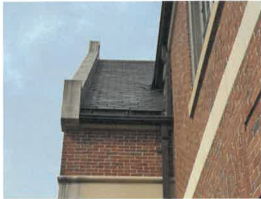
Fig. 36. Missing and loose slate.
