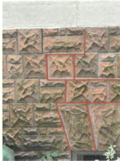
Fig. 7. Step crack through mortar joints. Red lines show locations of open or cracked joints.
