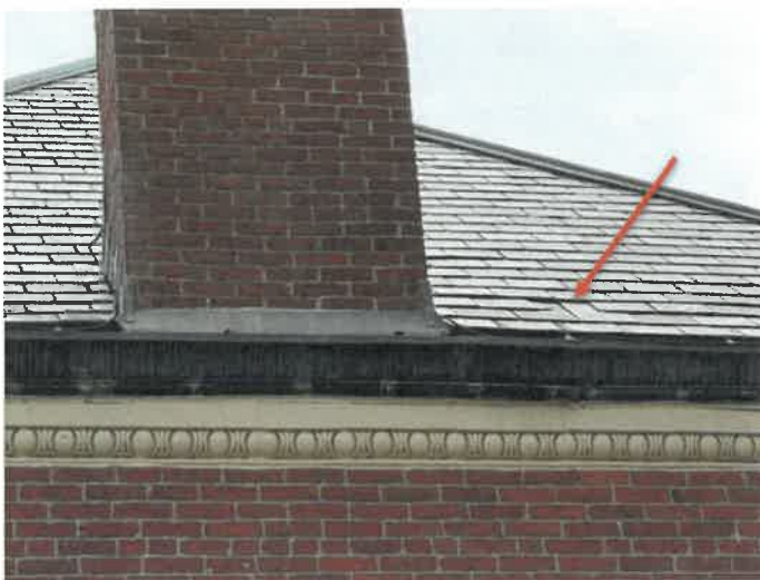
Fig. 9. Slate roof around west chimney showing loose and missing slate.
