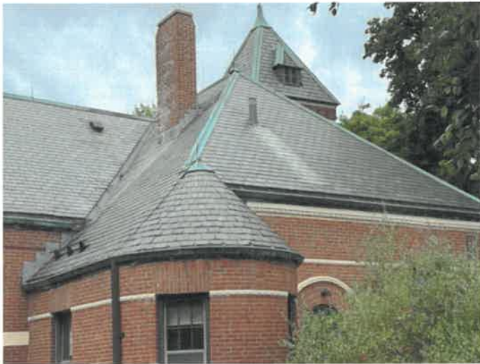
Fig. 10. Copper gutters, downspouts, valleys and hips.
