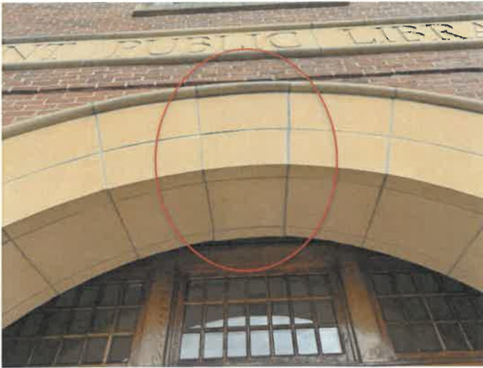
Fig. 29. Open mortar joints in arch.
