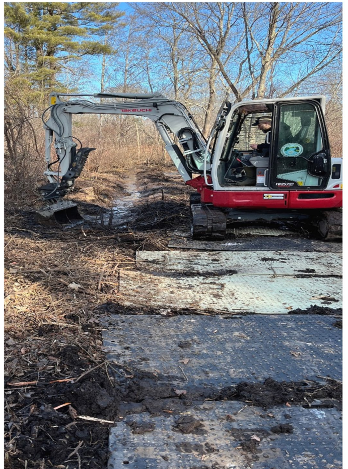
Image 6. Ground mats used to keep the area protected.
