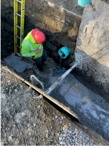
DeBush Avenue Water Main Installation
